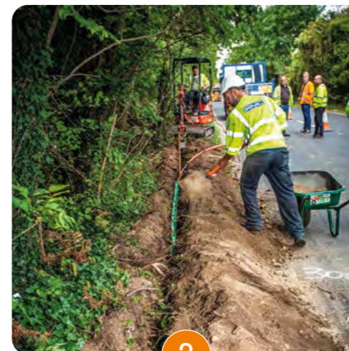
Trench is backfilled
