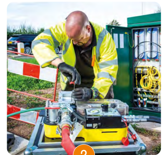
Fibre-optic cable is blown into ducting
